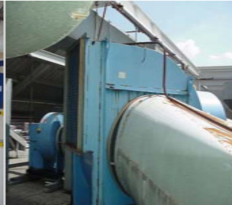
Exhaust fan with Rusty Ductwork
