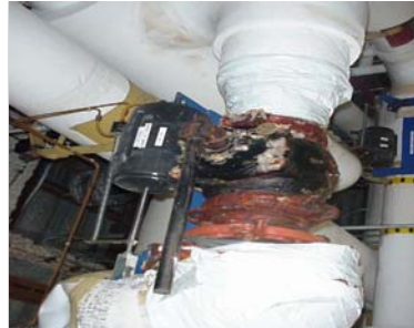
Corroded Valve
